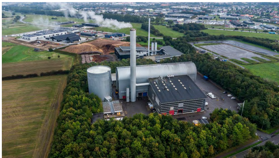
Sønderborg Combined Heat and Power Plant. The plant produces district heating and electricity through the energy recovery of non-recyclable residual waste. It is an important component of Sønderborg's collective heat supply, which COHEAT helped expand to additional households and communities, thereby supporting the replacement of individual oil and gas heating systems (Photo: Sønderborg Varme)
